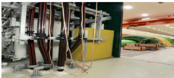
Figure 5: MMC based Motor Drive for a converter fed synchronous machine by ABB and Oberhasli Hydroelectric Power Company, Switzerland
