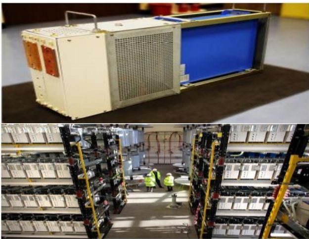
Figure 4: Sub-module (up) and MMC (down) structure of MaxSine
